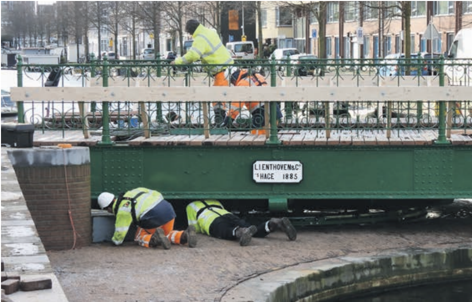
INSTALLATION OF THE BRIDGE DECK
