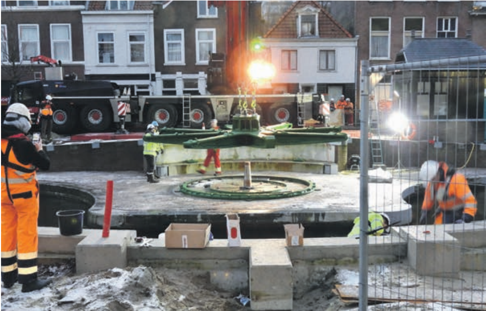
THE SPIDER, THE ROTATING PART OF THE BRIDGE.
